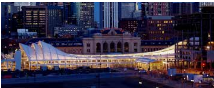
Denver Union Station / Denver, CO USA
