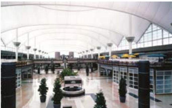
Denver International Airport
